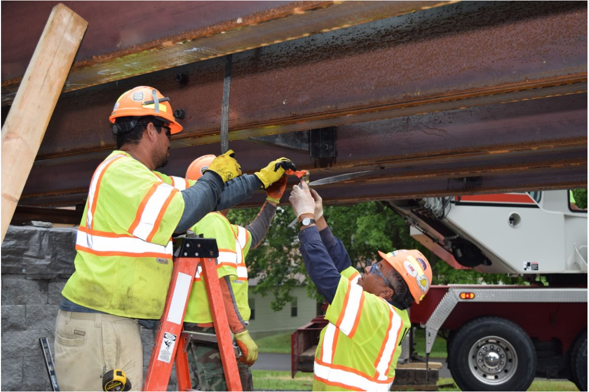
Workers prepare to transport bridge components
