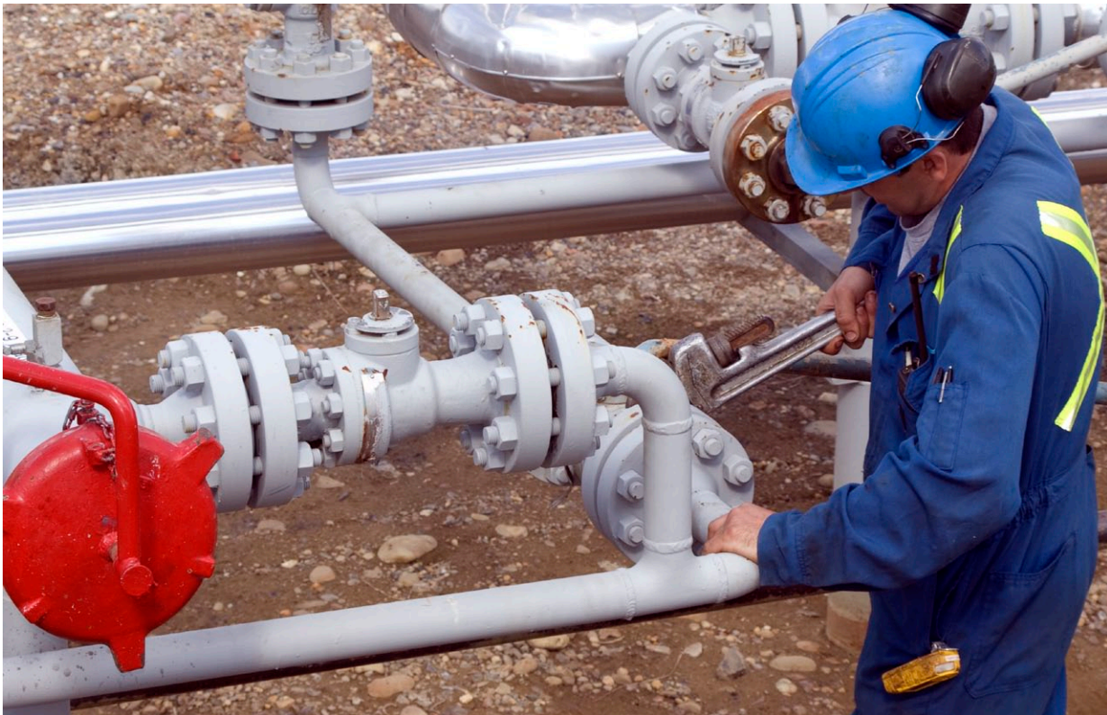
Repair and testing of pipeline infrastructure during a safety review
