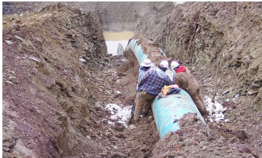
Workers near excavated pipeline
