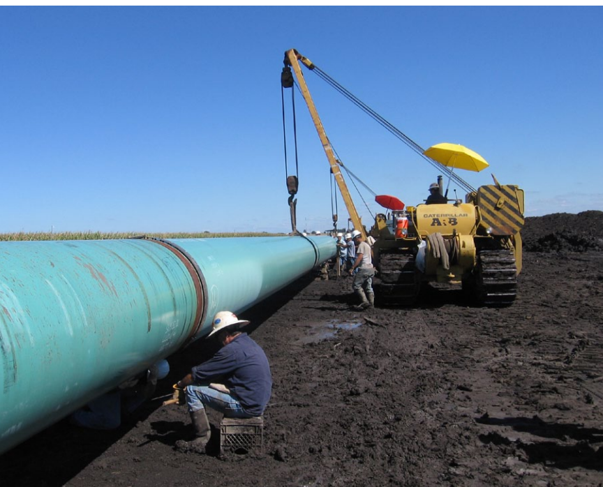
New pipeline under construction
